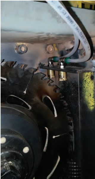
Rip saw installation.
